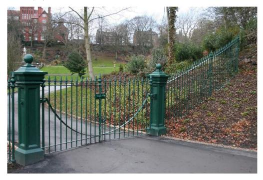
The Ivy Bridge gates shown below not only feature the conical topped railings but also include distinctively shaped urns, produced in cast iron to replicate those shown on original photographs of the installation but missing by the time of the restoration project.
