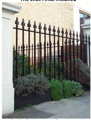
The Eliot finial, produced from the Lost Art pattern and installed in the conservation area of Liverpool.
