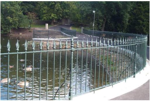
The railings surrounding the park include fleur-de-lys finials in a variety of sizes, some lead set into the copings of the perimeter wall, with others assembled into separate panels and installed between supporting posts. All the new railings were produced and then installed by Lost Art Limited
