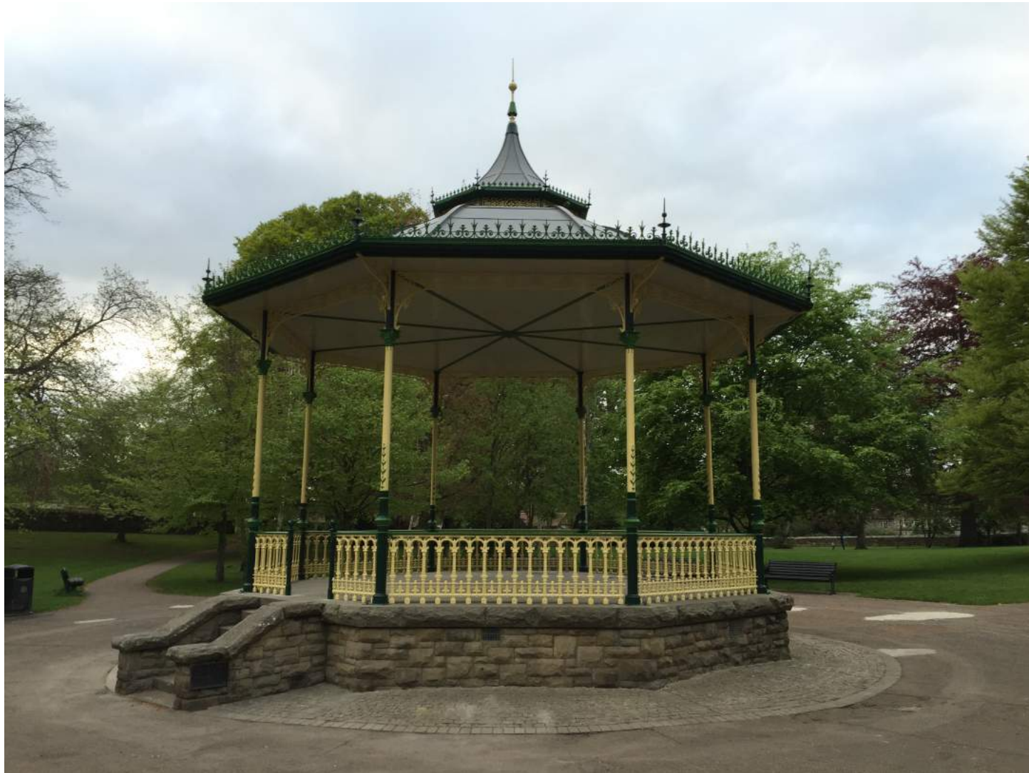
Hexham: Sele Park: Full Restoration
