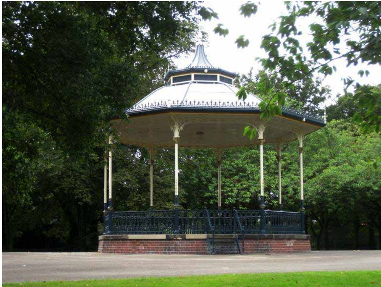
East Park, Wolverhampton: Full restoration
